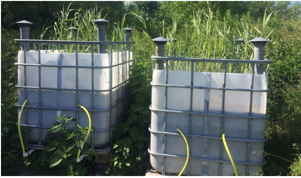
Constructed pilot plant of RBS at WWTP in Swarzewo: two cubic pilot plants RBS (August 2020), photo: A. Kupczyk
