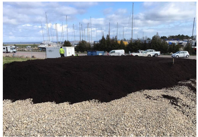
Construction of the biocover at Tangmoseskoven in 2020.
